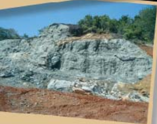
blasting through rock
