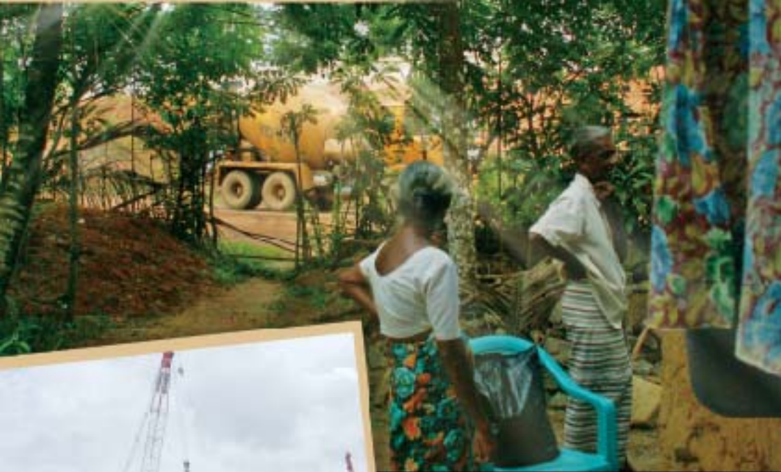
construction close to house
