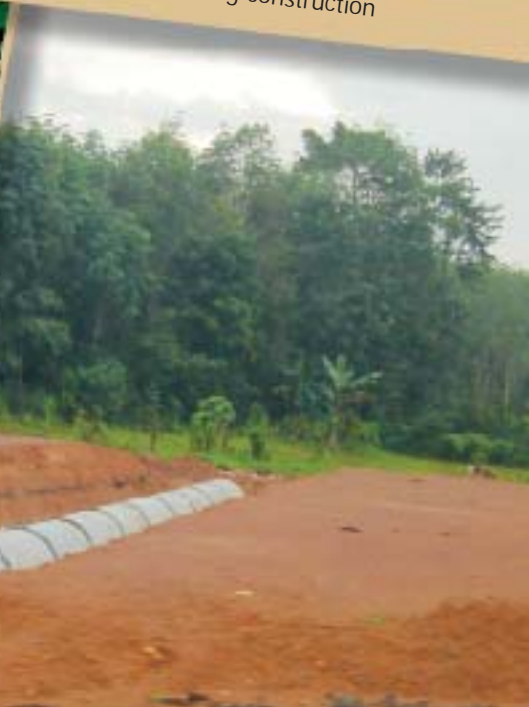
water pipe in highway
