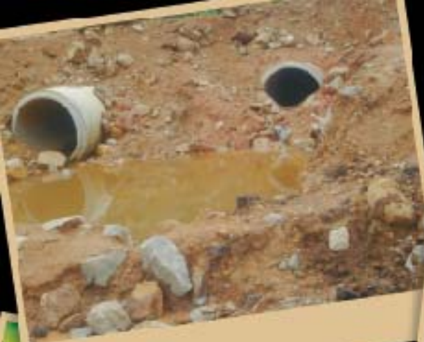
constructing culverts
